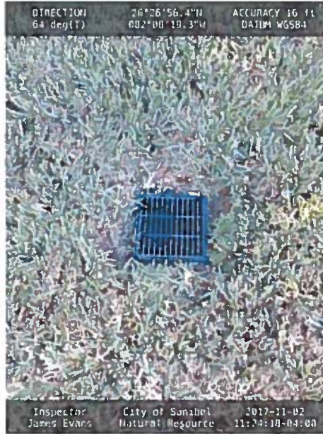
Figure 3 Photo of underdrain in stormwater swale located at 4702 Rue Belle Mer.
